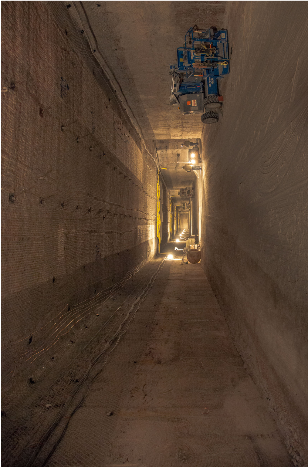
Figure B4-2 Underground - Panel 7 - Panel Entry
