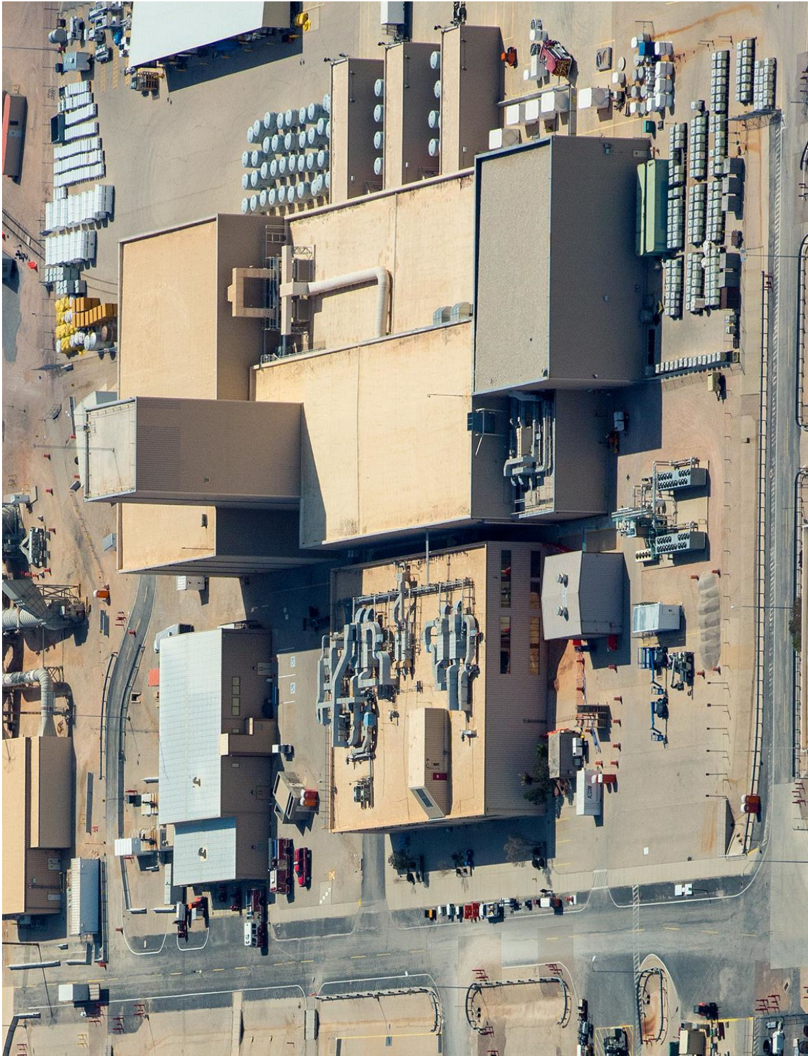
Figure B4-3 Aerial Photograph of the Waste Handling Building
